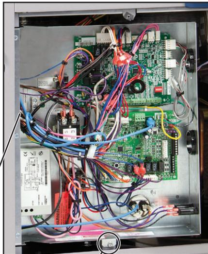
Ground Fastener must be installed for proper unit ground
