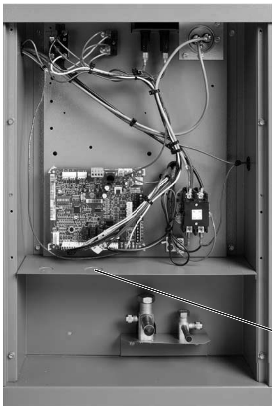
Figure 13A: Wire access (control box open)
