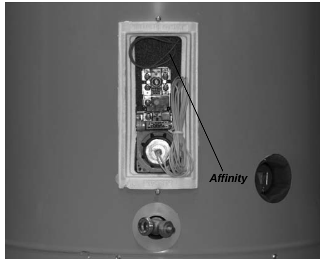
Thermistor Wires Connected to TB (3 and 4) on Affinity Series Control Board
